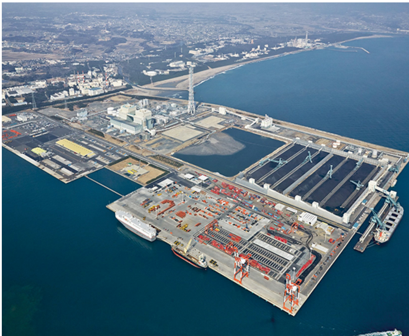
Hitachinaka Thermal Power Station
